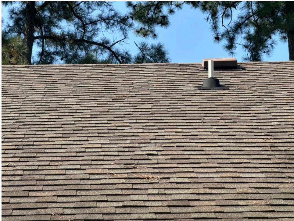
Roof verification, Rear, Left, Roof
