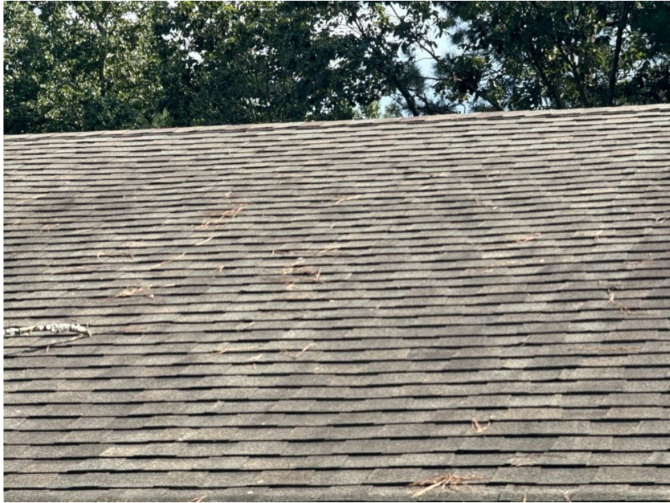
Roof verification, Rear, Right, Roof
