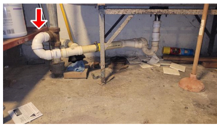
3.4 Under laundry tub
