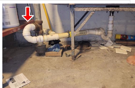
3.4 Under laundry tub
