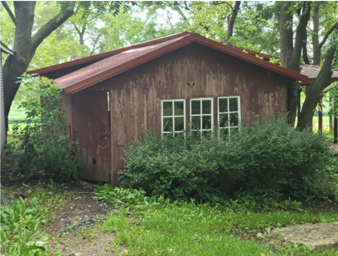
27 Detached Structure Hazard
