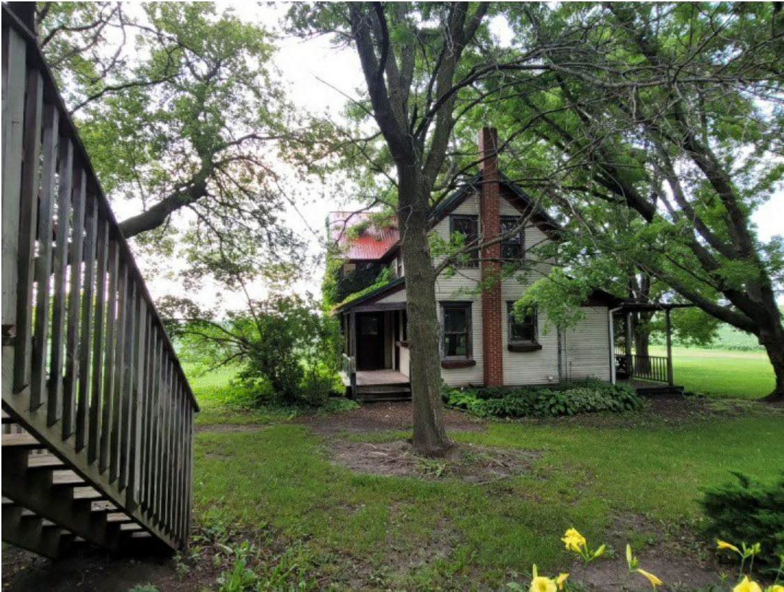
34 Detached Structure Hazard
