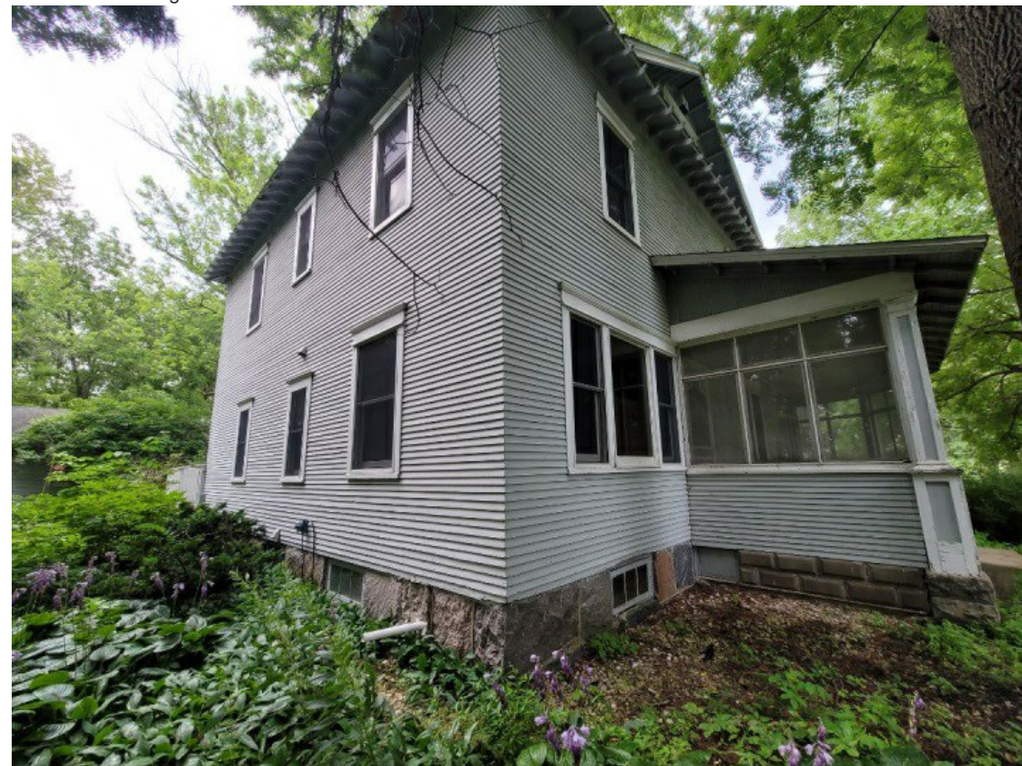
20Left Rear of Dwelling
