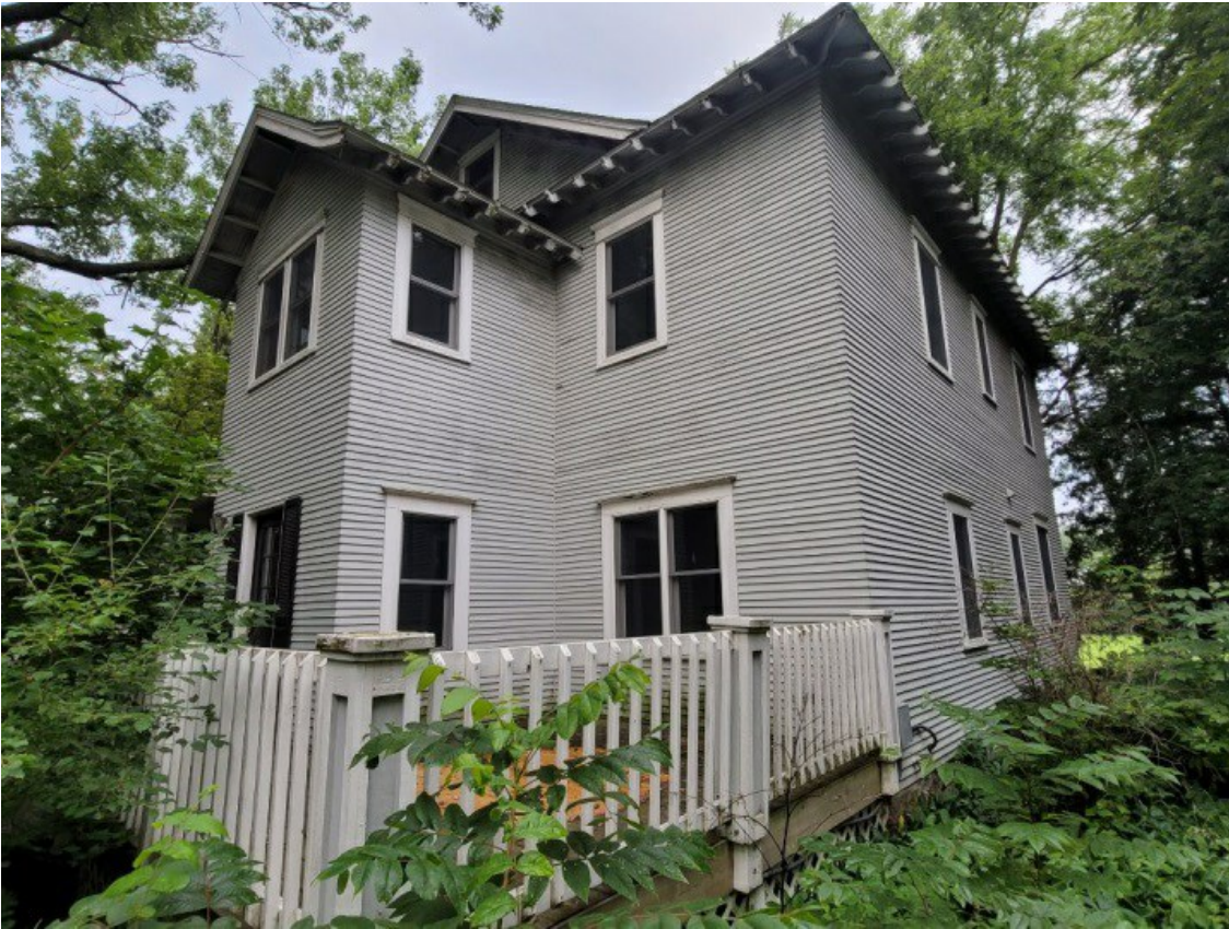
16 Right Rear of Dwelling
