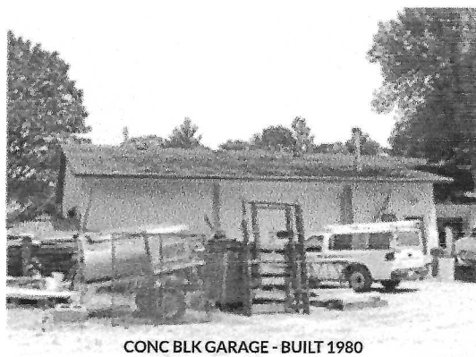
CONC BLK GARAGE - BUILT 1980
